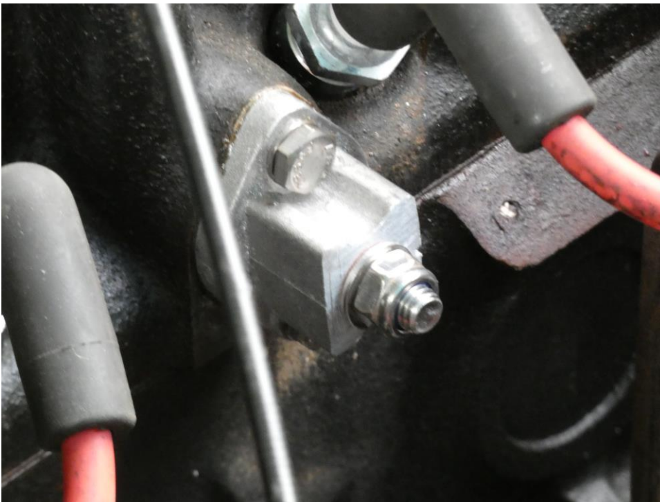
↑ It doesn't look too bad.
